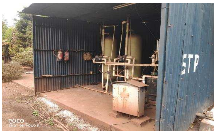
Photo-8: STP for treatment of Domestic Waste Water (Ultra Filtration Unit) & its utilization in green belt development
