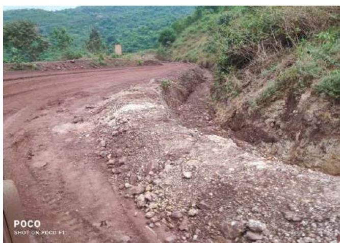
Photo-4: Showing Check weirs, Settling pond and Garland drain
