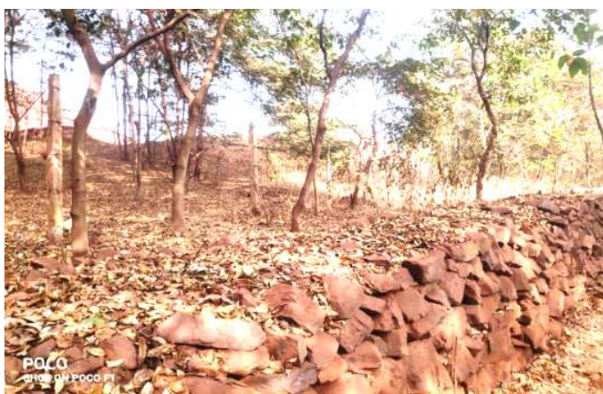
Photo-5: Retaining wall at toe of dumps
