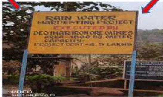
Photo-12: Roof top Rain Water Harvesting structure & Recharge pit
