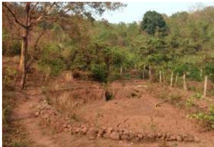
Photo-8& 9: Settling cum water harvesting pit
