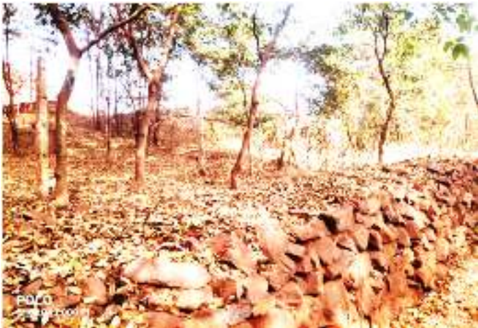
Photo-2 &3: Retaining wall along with Plantations at the toe of dump slopes
