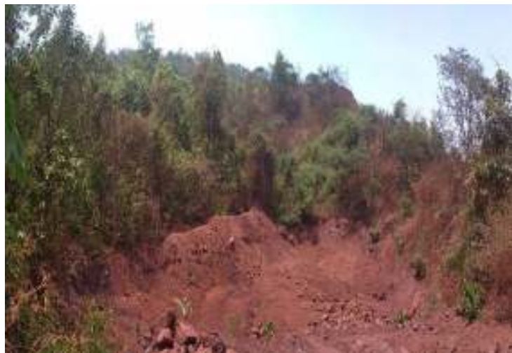
Photo-8& 9: Settling cum water harvesting pit
