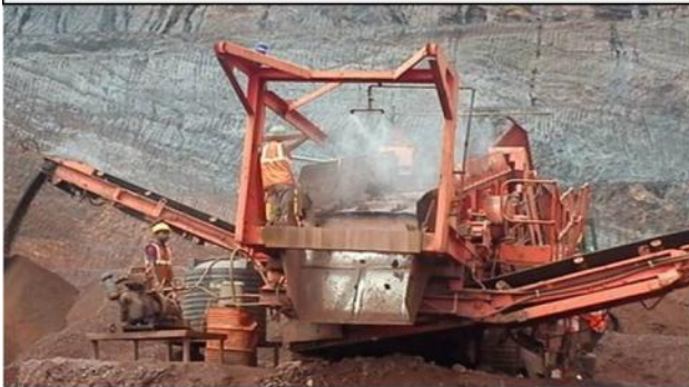
PHOTO # 1-B SHOWING THE CRUSHER & SCREEN PLANTS ENCAPSULATED WITH HOODS AND DRY FOG SYSTEM
