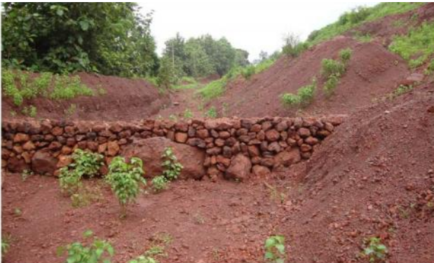
PHOTO # 2 SHOWING CHECK WEIRS AT DIFFERENT STRATEGIC POINTS
