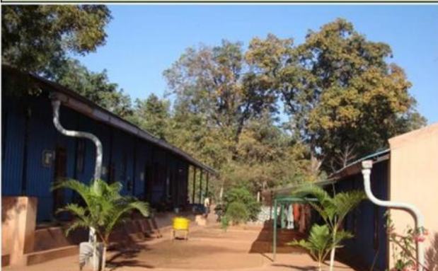
PHOTO # 5 : SHOWING RAIN WATER HARVESTING STRUCTURE FOR GROUND WATER RECHARGE @ CAMP AREA
