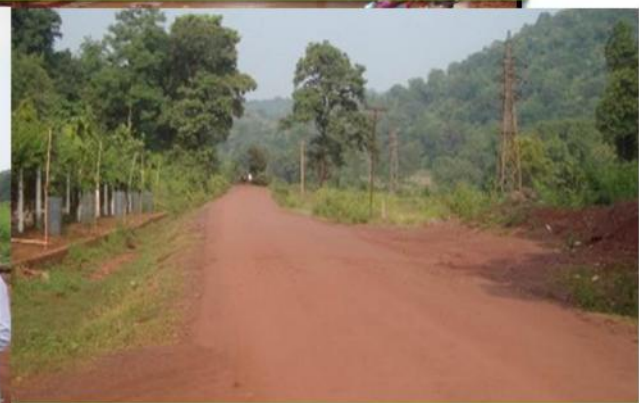
PHOTO # 14 SHOWING BLACK TOPPING OF VILLAGE ROAD
