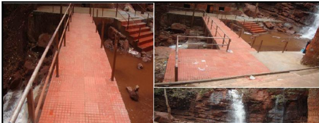
PHOTO # 15 SHOWING MAHA DEV NASA TEMPLE RENOVATION WORK
