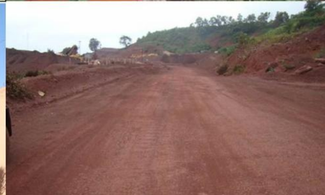
PHOTO # 4: SHOWING HAULAGE ROAD MAINTENANCE BY GRADER
