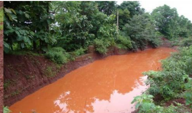
PHOTO # 3: SHOWING SETTLING PIT BEFORE FINAL DISPOSAL TO OUTSIDE WATER BODIES
