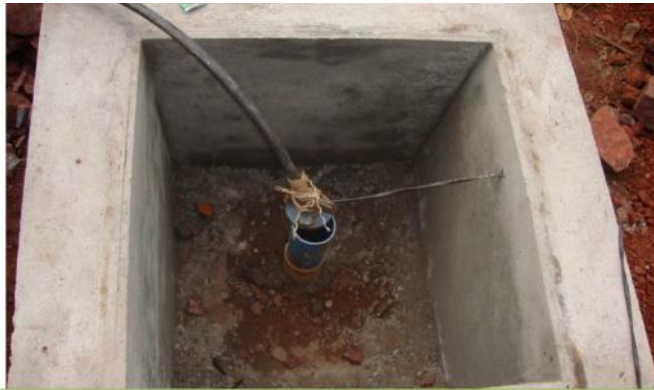
PHOTO # 13 SHOWING BORE WELLS PROVIDED FOR VILLAGERS
