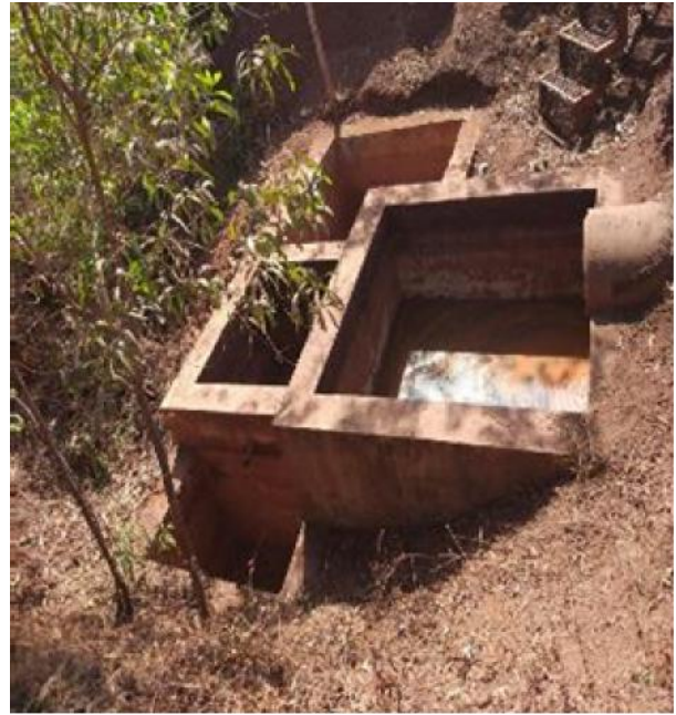
Pic 10- Effluent Treatment Plant
