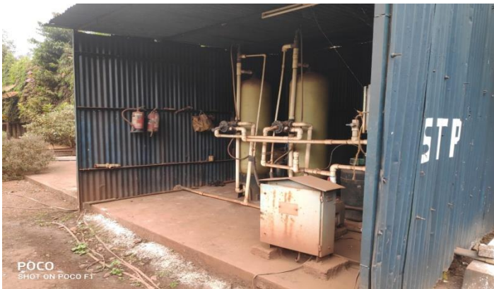
STP at staff campus and use of treated water for green belt development
