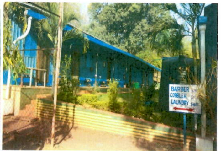
Rain Water Harvesting
