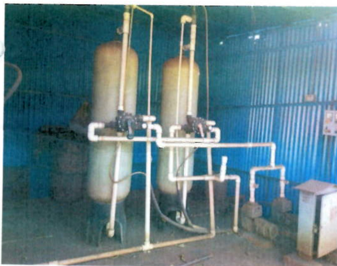
Sewage Treatment Plant
