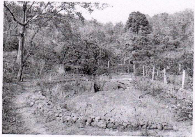
Settling cum water harvesting pit
