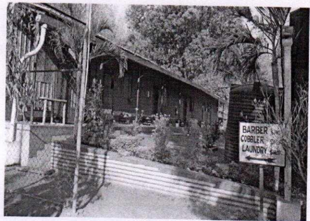
Roof top Rain Water Harvesting structure
