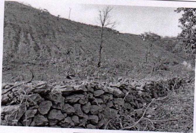
Retaining wall along with Plantations at the toe of dump slopes
