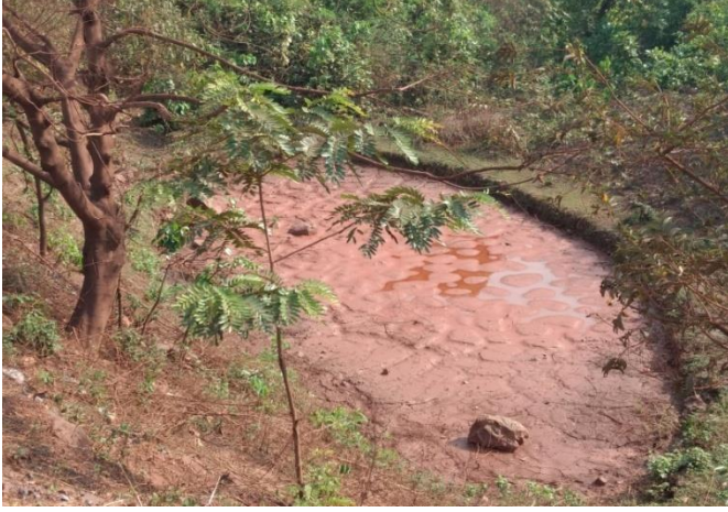
Settling cum water harvesting pit
