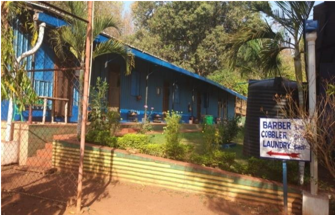
Roof top Rain Water Harvesting structure
