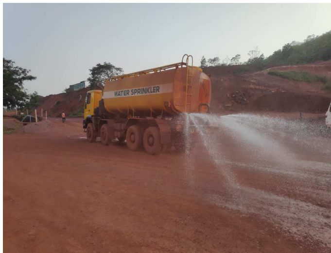
Water sprinkling with mobile water tanker
