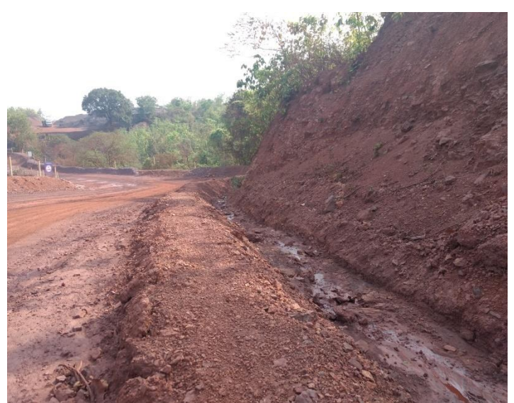
Photo showing Settling pit, Check weirs, retaining wall & earland drain
