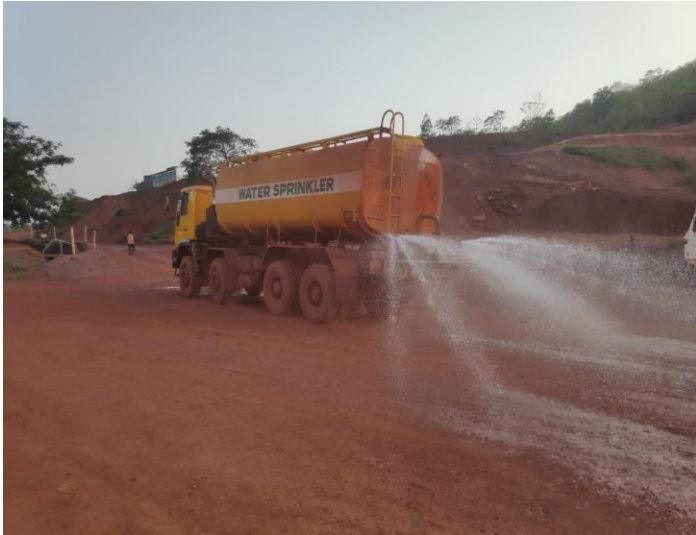
Water sprinkling with mobile water tanker
